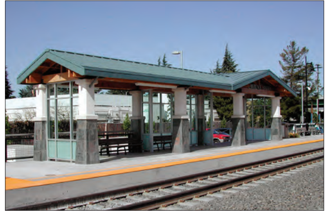
▲ Figure 3: A rail station can function with just a platform, ticket kiosk, and surface parking lot. However, a well-planned rail station can become a valuable community asset.
