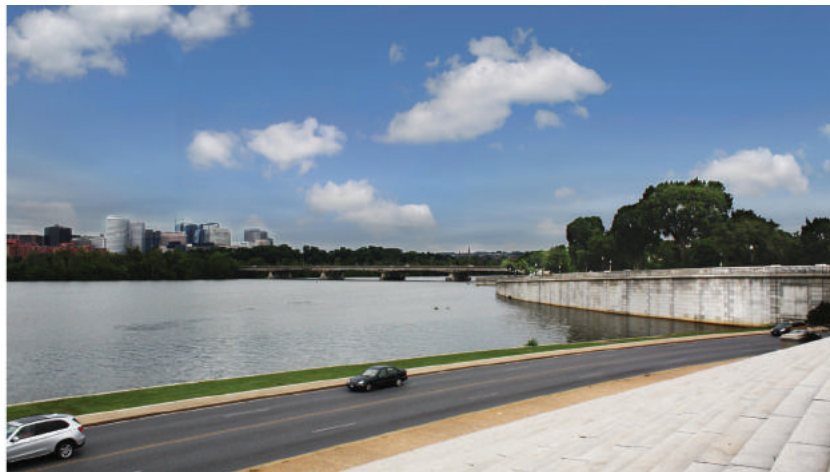
2 Ohio Drive Steps
