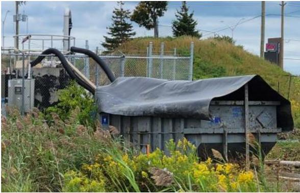
Figure 5 Biofilter
