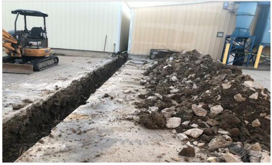
The "trench" is about 20 inches deep, and we had buses parked on both sides to stop traffic going around the bus barn to music room. It has been filled in with cement at this time and is open for traffic again.
