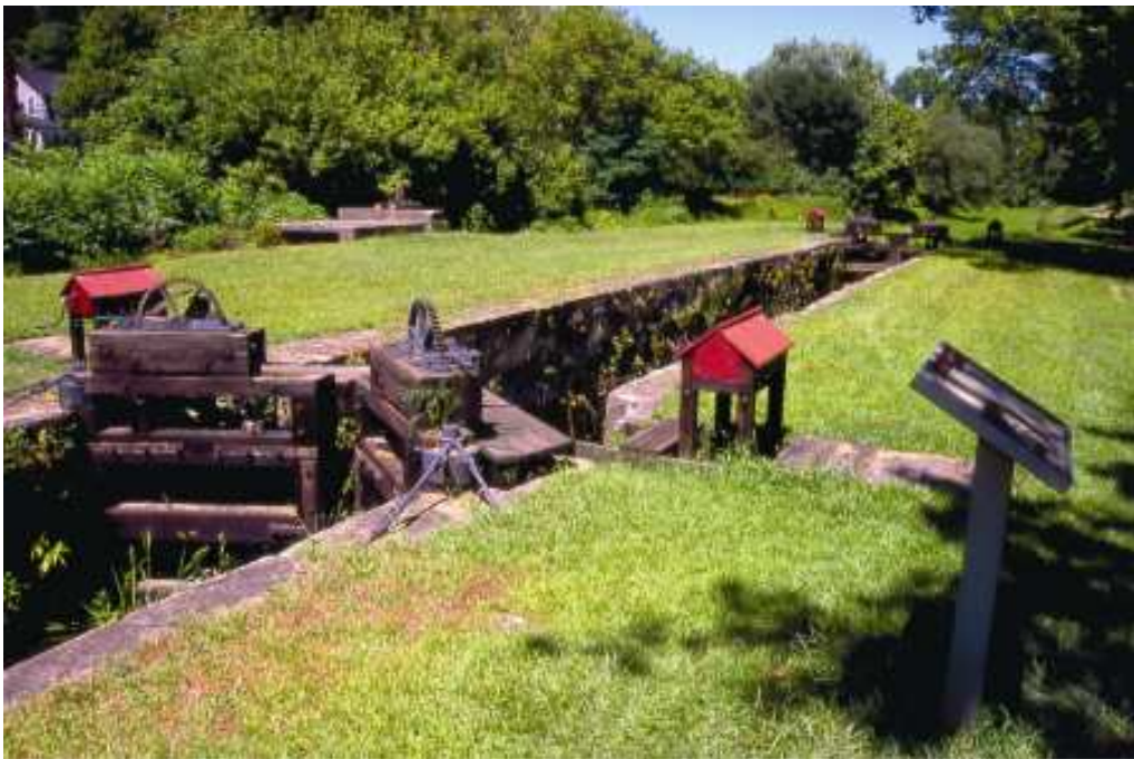
A low-profile sign interprets the remains of Lock 21 in Delaware Canal State Park.
