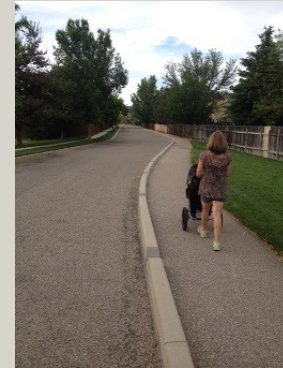
Extruded curb and shoulder space can improve safety with minimal investment.
