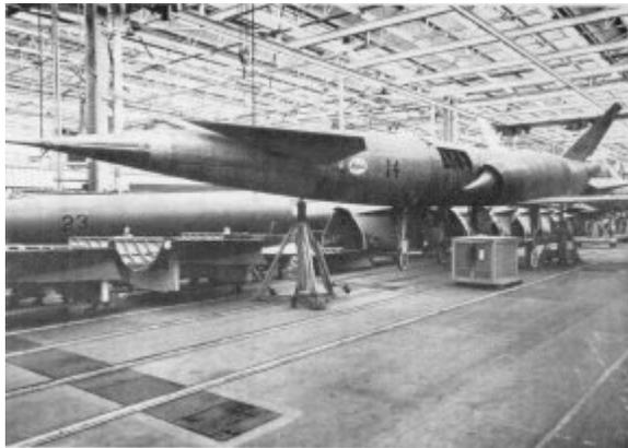
**Photo from the James Gibson Collection G-26 Vehicle No. 14 being completed at the Downey facility. The jack placed under the guidance section kept the vehicle level during assembly. Otherwise, the short nose gear would make the nose droop. The tails of the missile were so high, the main landing gear had to be retracted and the missile pulled out on a low dolly. The four foot diameter ramjets are the largest to have ever flown to this**
