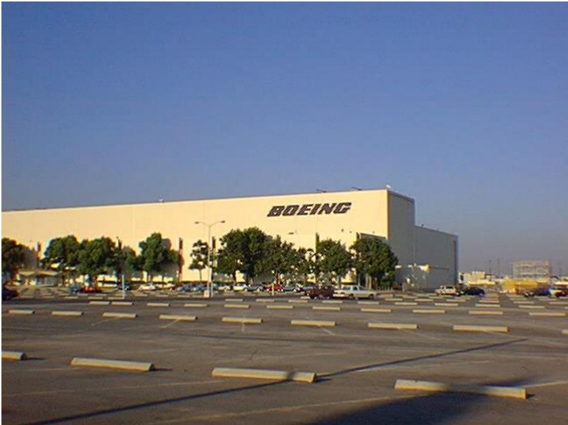
The building was designed and constructed in 1964. It consists of a two-story structure of concrete and steel beams with a flat roof on the west side. A High Bay section (80 foot ceiling), a Low Bay section (40 foot ceiling) and a two story section east of the low bay adjacent to Building 6. The total square footage is 165,100.
