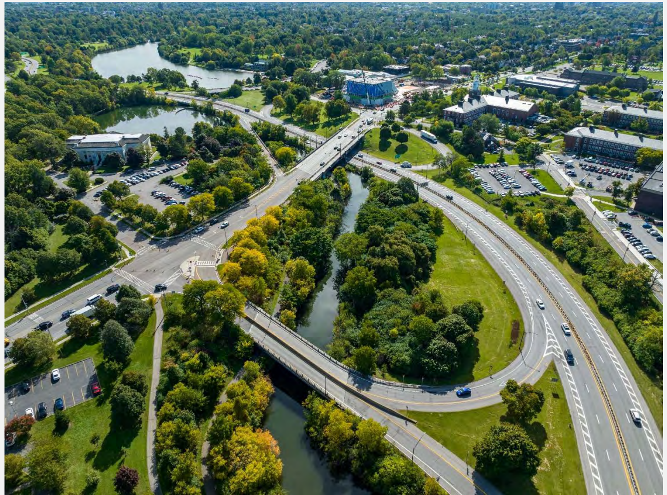
Scajaquada Expressway crossing Scajaquada Creek. Source: Stantec
