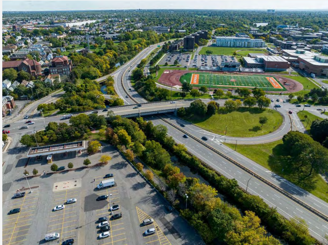
Scajaquada Expressway looking east over Grant Street. Source: Stantec.
