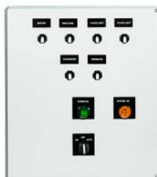
HELIPORT LIGHTING CONTROLLER PHC-61001-1-SC1
