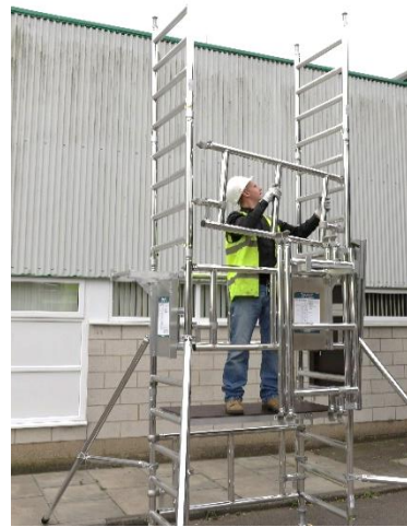
23. Retrieve a side guardrail frame from the front assembly bracket and locate it as shown.
