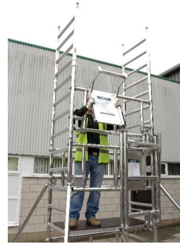
24. Relocate the side "empty" assembly bracket on the front of the tower (top rung of the tallest guardrail frame as shown)
