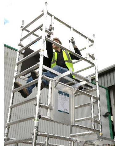
28. Fit 2 guardrail frames, with the top hook (facing outwards) set above the top rung of the frame.
