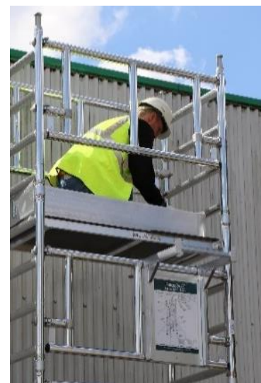
14. Fit toeboard by unfolding the set above the platform (please use labelling as a reference to ensure that the toeboard is the correct way up).
