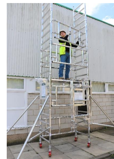
20. Fit 1 side guardrail the 3 rd rung above the existing as shown.
