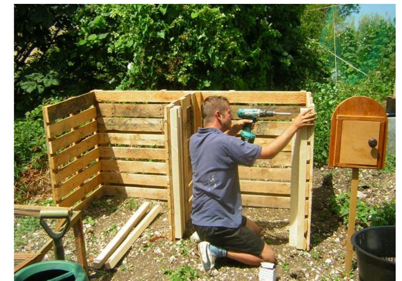
Local joiner making pallet compost bays
