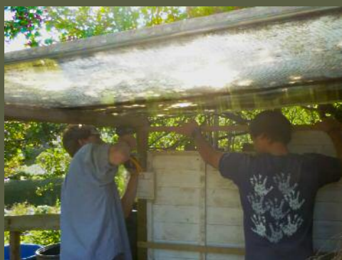
Local lads built a storage area using donated shed panels in an afternoon.
