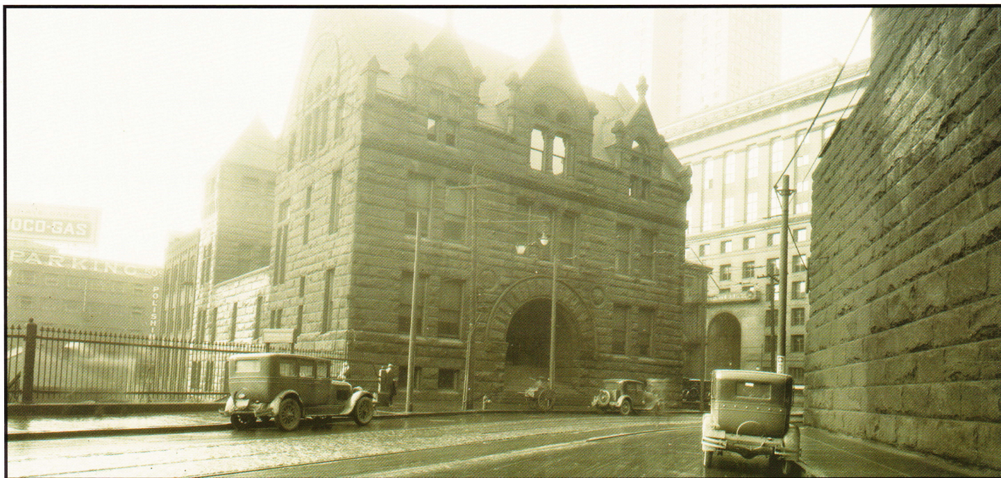
Allegheny County Mortuary, Fredrick Osterling; Built 1902; Moved in 1929; 604 Fourth Avenue, Pittsburgh
