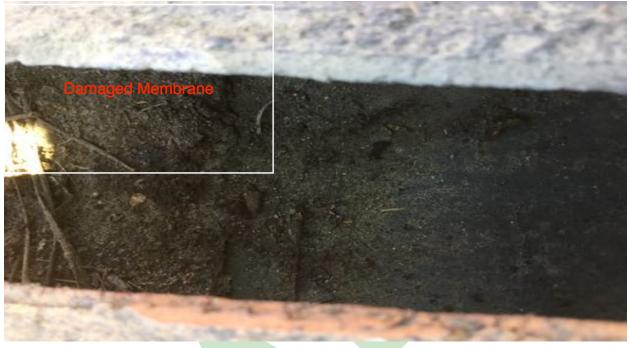
REPLACE – SHOWN BELOW IS THE DETERIORATED MEMBRANE UNDERNEATH CLAY TILE SYSTEM. MEMBRANE CURRENTLY HAS CRACKS AND IS DRY TO TOUCH. MEMBRANE IS COMPOSED OF 15 POUND TAR UNDERLAYMENT THAT IS OUTDATED AND IS CURRENTLY FRAGILE. MEMBRANE PROVIDES NO WATERPROOFING AND IS CRACKED IN MULTIPLE LOCATIONS. RUSTED FLASHING IS SHOWN BELOW WITH CRACKING THROUGHOUT.
