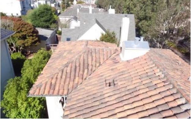
REPLACE – SHOWN BELOW IS THE MEMBRANE OVER FLASHING AT ONE OF THE ROOFING VALLEYS OF THE ROOFING SYSTEM. MEMBRANE IS CRACKED EXPOSING FLASHING SYSTEM. FLASHING SYSTEM IS MADE OUT OF GALVANIZED STEEL AND IS RUSTED IN MANY LOCATIONS PROVIDING NO WATERPROOFING.
