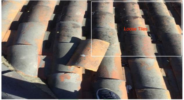
REPAIR – SHOWN BELOW ARE THE CRACKED CLAY TILES AT THE EDGE OF THE ROOFING SYSTEM AND CLOGGED GUTTER WITH NEGATIVE SLOPE THAT HAS STANDING WATER INSIDE ALONG WITH DEBRIS AND DIRT.
