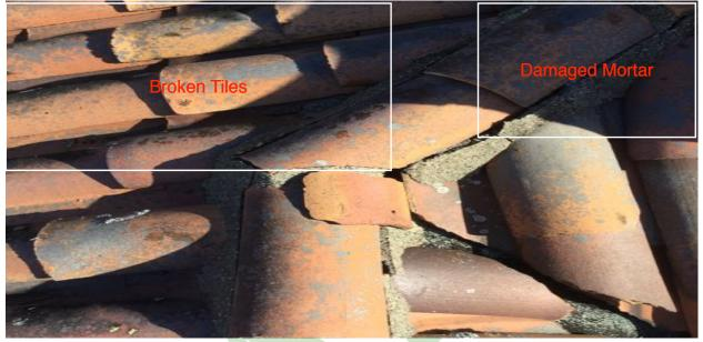
REPLACE - LOCATED THROUGHOUT ROOFING SYSTEM, MORTAR LINES BETWEEN CLAY TILES HAVE FAILED AND HAVE SHIFTED PRESENTING WATERPROOFING ISSUES AND A RISK OF INJURY IF SEPARATED COMPLETELY.
