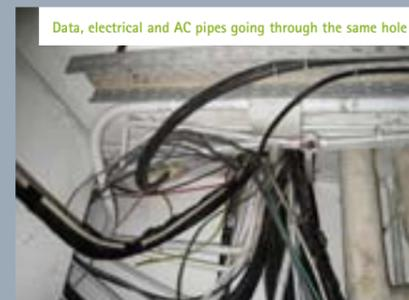
Data, electrical and AC pipes going through the same hole
