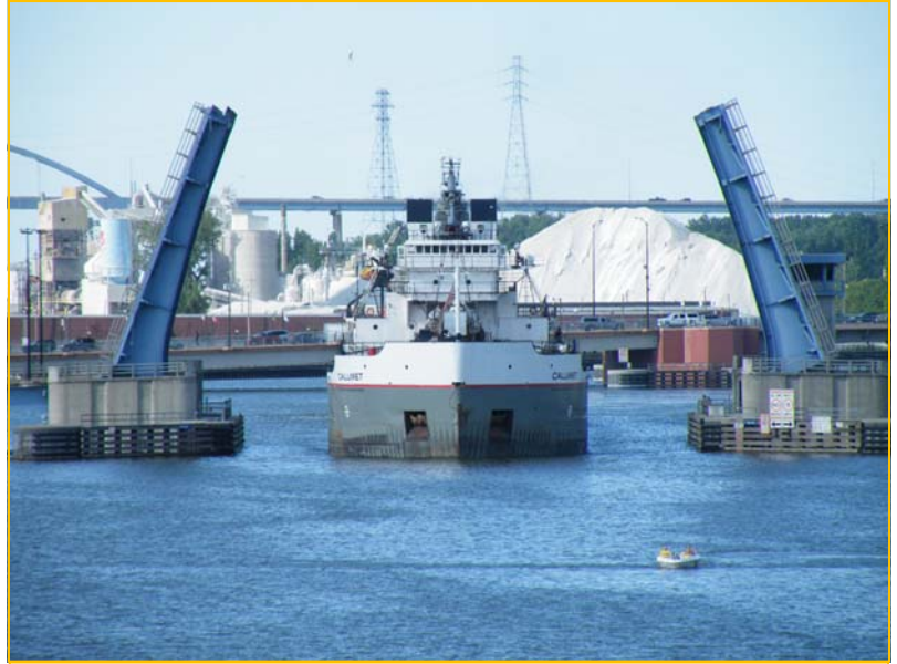
Manitowoc traveling through the Main St. Bridge
