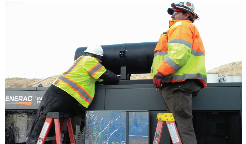
Christopher Wippel & John LaFountain, Electricians
