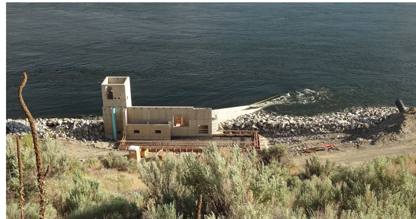
Fish ladder and broodstock "fish elevator" is nearing completion.
