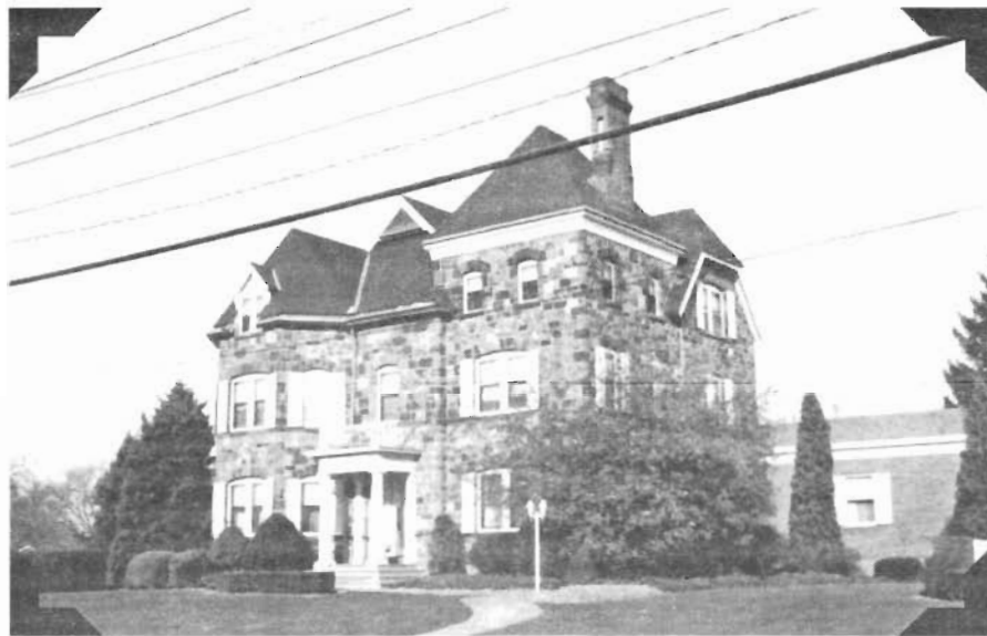
The stately Richardson Romanesque stone building at the corner of Springfield and Morris avenues that was for many years Brough Funeral Home is being converted to become the centerpiece of a large office building. For many years, it was the home of William Risk, who with his brother James is credited with helping to found and support many of the organizations and services that helped Summit become the city it is today.
