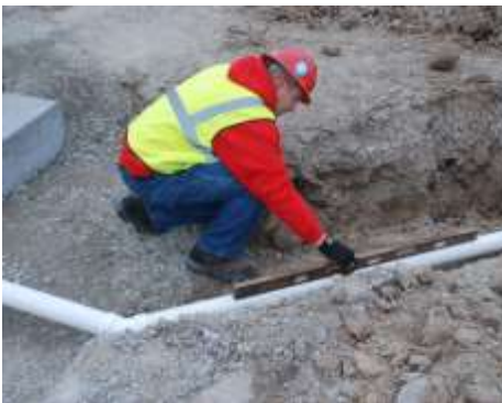
Step 7: Slope 4 inch PCV drain away from foundation and run 1" conduit from scale to controller
