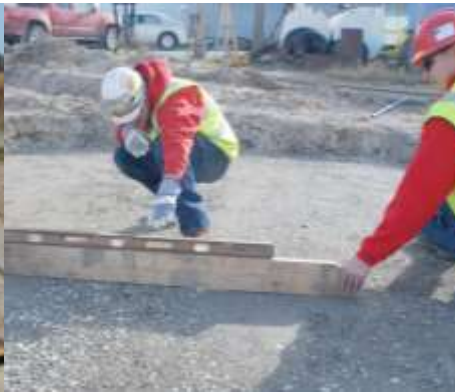
Step 5: Entire foundation must be flat and level. This is the most critical step toward achieving accuracy
