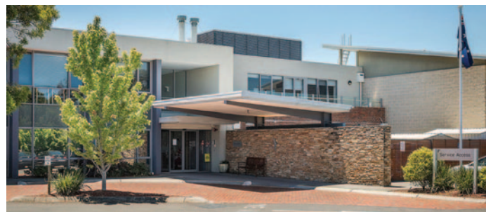
The refurbished VMCH Corpus Christie Aged Care Residence in Melbourne. All photos: Michelle Despot from M Style & Co
