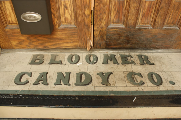
Mosaic Tile in the entryway to the former Bloomer Candy Co building on N 3rd St. which is expected to be demolished for make room for a parking lot.
