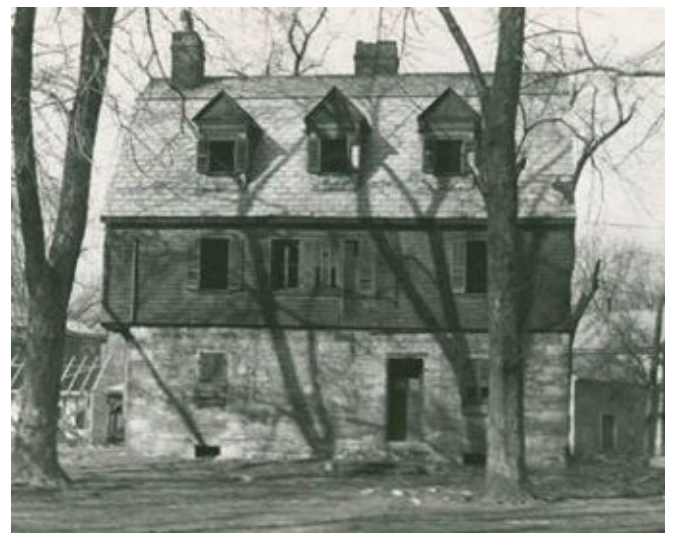
The Dr. Increase Mathews House before it was preserved by William Adams in 1937. Without his work, this would likely be a vacant lot today.
