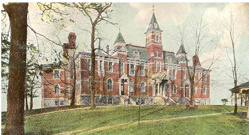
The McIntire Children's Home stood on the grounds of the present Zanesville High School from 1880 until 1944.
