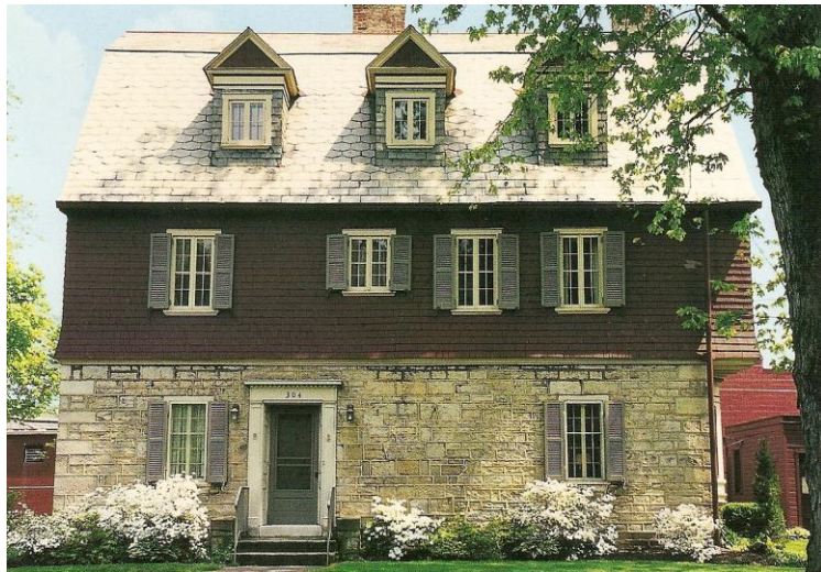
Dr. Increase Mathews' house as it appears today. The upper two stories were added after the doctor's death. Photo by Stephanie Kline.
