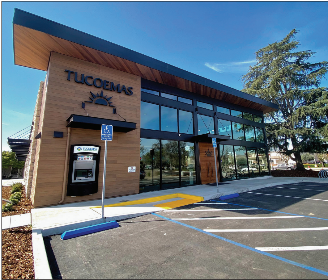
Tucoemas Federal Credit Union earned a gold certificate for environmental design at their new flagship Akres branch in Visalia.
