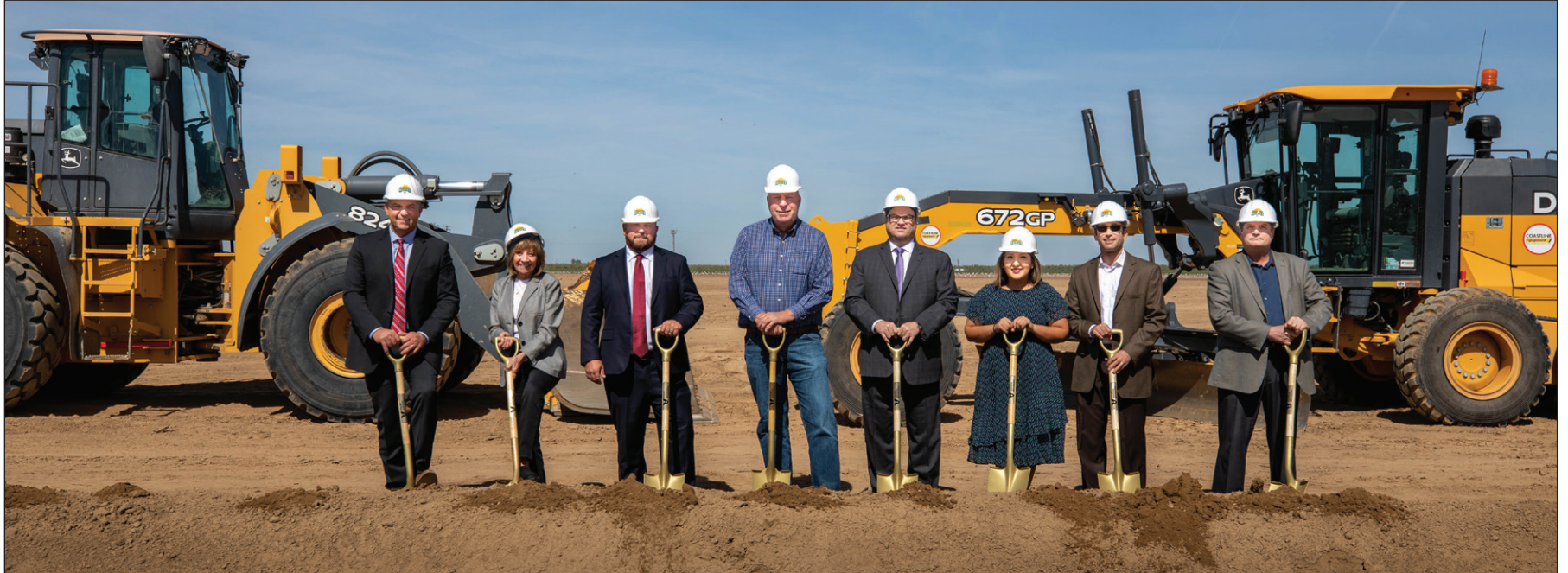
California Dairies, Inc. broke ground on their soon-to-be facility partially powered by renewable energy.
