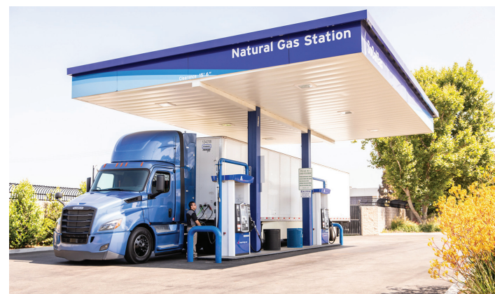
PHOTO COURTESY SOUTHERN CALIFORNIA GAS COMPANY In 2020, SoCalGas began dispensing California-produced renewable natural gas (RNG) at many of the natural gas fueling stations it operates across the state.
