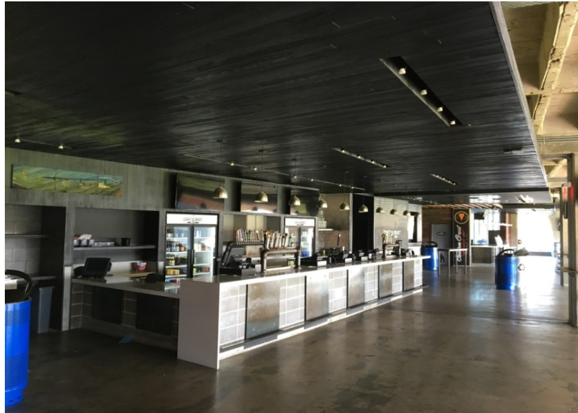
Figure AI-8: Wood Plank Ceiling at Craft & Draft Area
