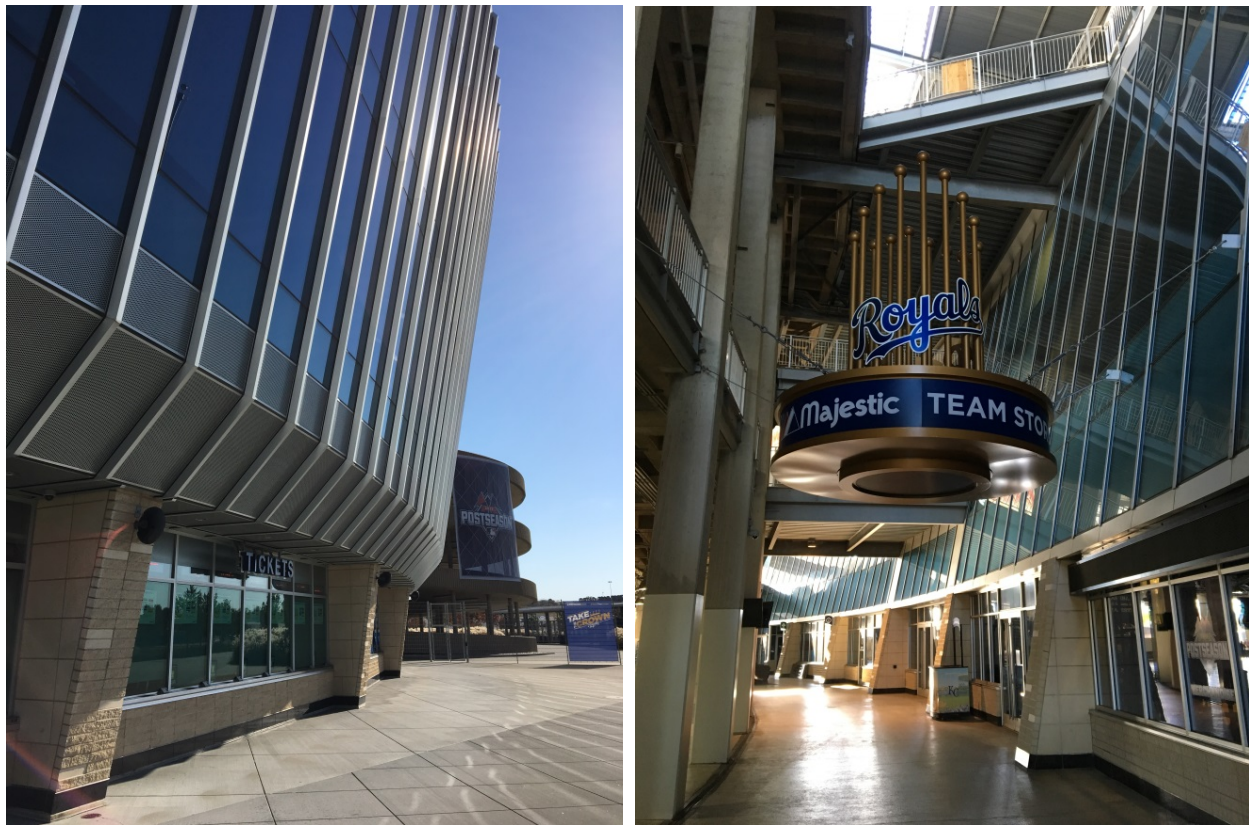
Figure AF-2: External (left) and Internal (right) Storefront, Curtainwall, and Stone Veneer
