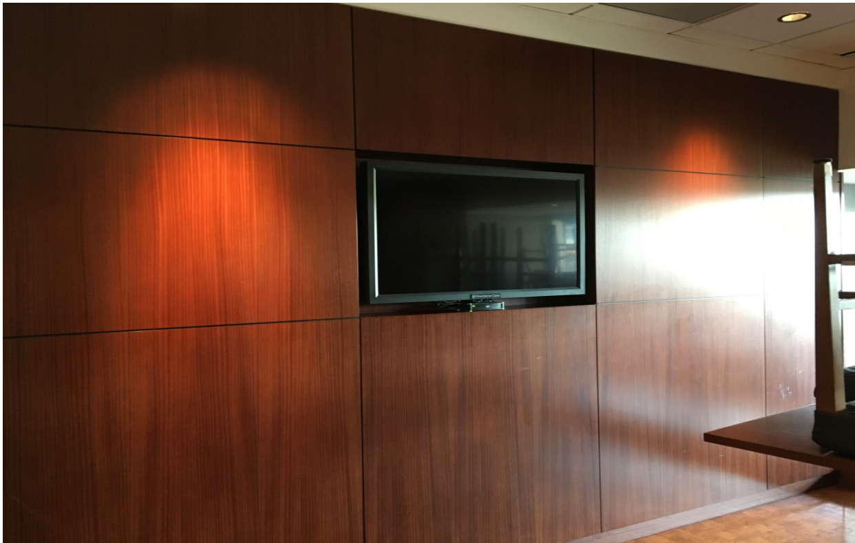
Figure AI-4: Wood Veneer Panel Wall
