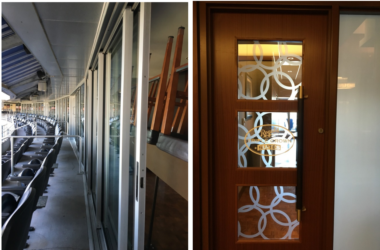
Figure AI-11: Typical Sliding Glass Wall System (left) and Wood Framed Glass Door (right)
