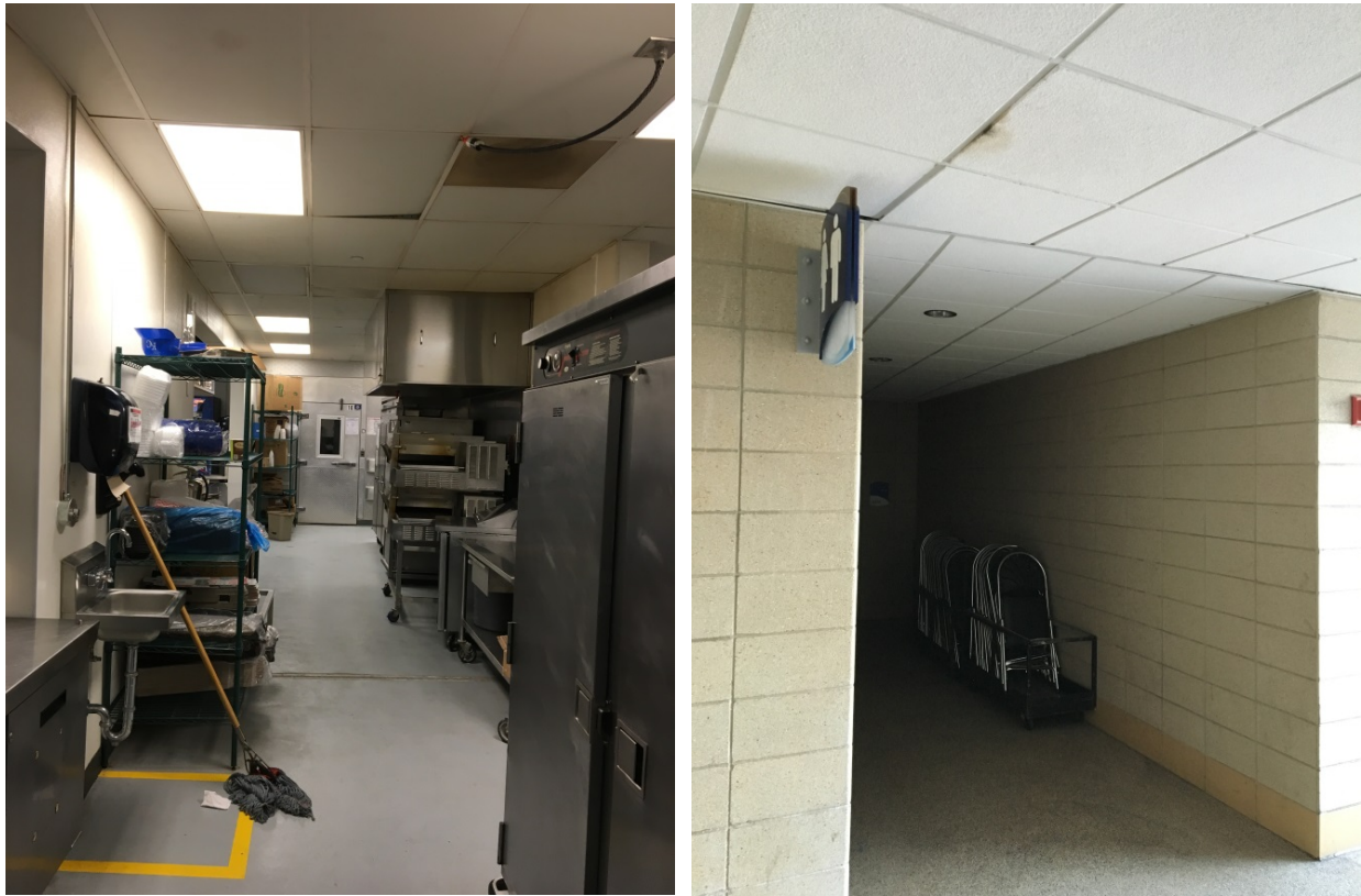
Figure AI-7: Interior and Exterior Acoustical Ceiling Tiles
