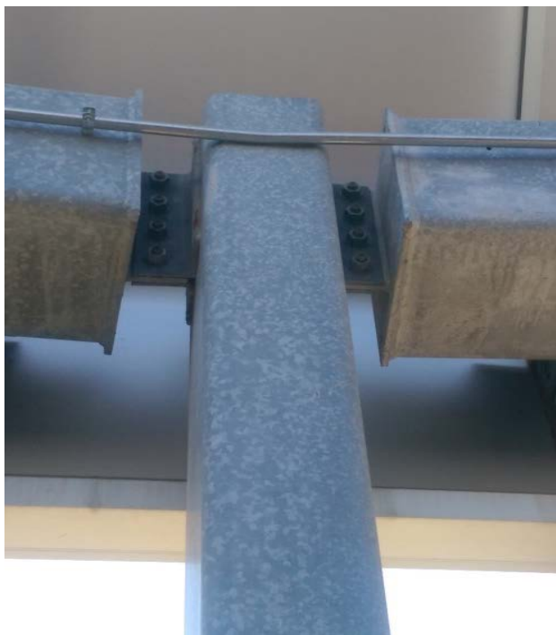
Figure S-3: HSS Beams, Column and Connections
