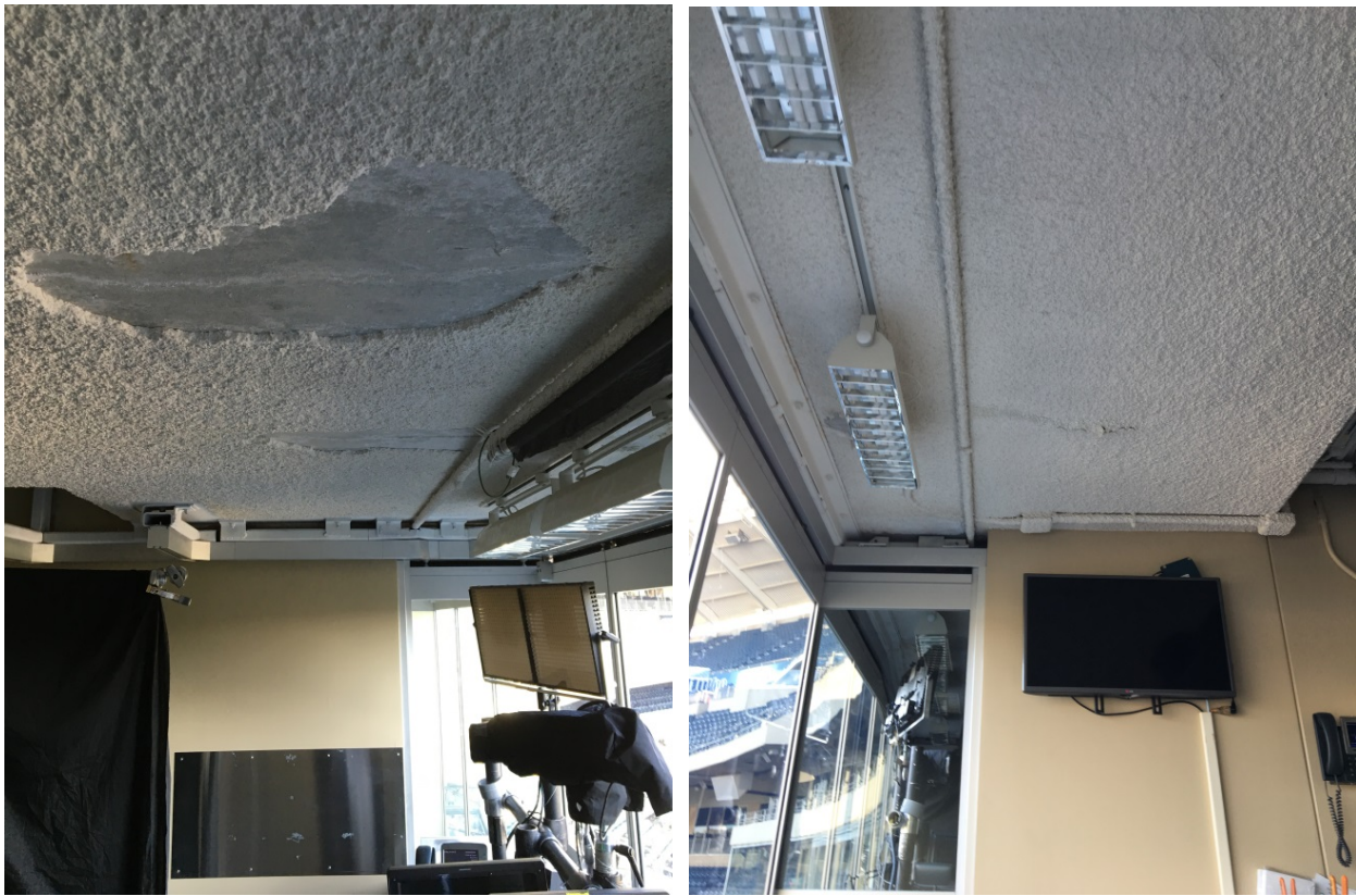
Figure AI-5: Sprayed on Fire Proofing at Exposed Concrete Structure
