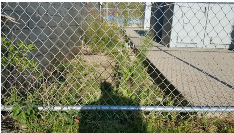
Figure L-5: Vegetation and Sedimentation indicate potential Water Ponding in this Area
