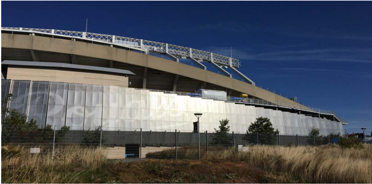
Figure AF-3: External Perforated Metal Panel System
