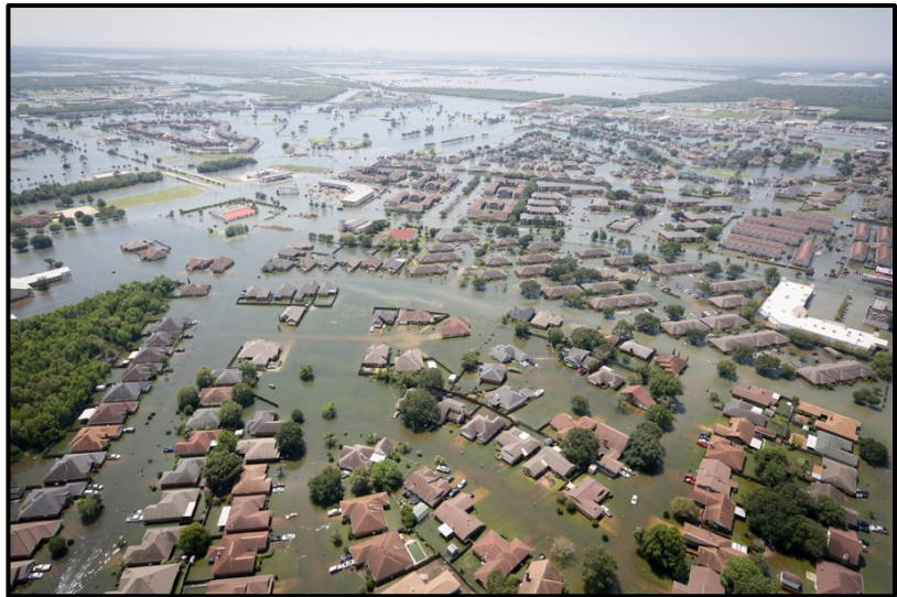
Figure 8: Flooding in Port Arthur, Texas on August 13, 2018 after Hurricane Harvey.
