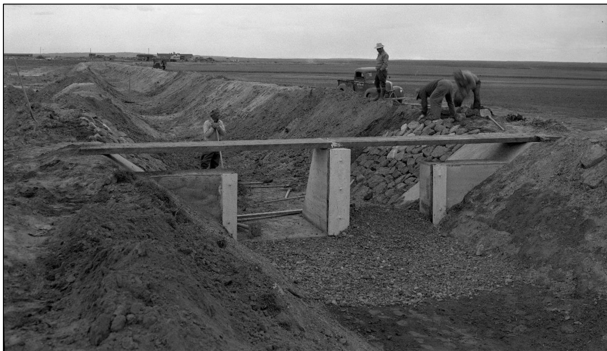
Figure 24: Irrigation ditch construction near the Minidoka concentration camp. Image available at the Densho Digital Repository, Object ID: ddr-fom-1-805 (NARA ID: 210-CMA-IC-6), Parent Collection: War Relocation Authority, Minidoka Collection, https://ddr.densho.org/ddr-fom-1-805/ . Courtesy of the National Archives.
