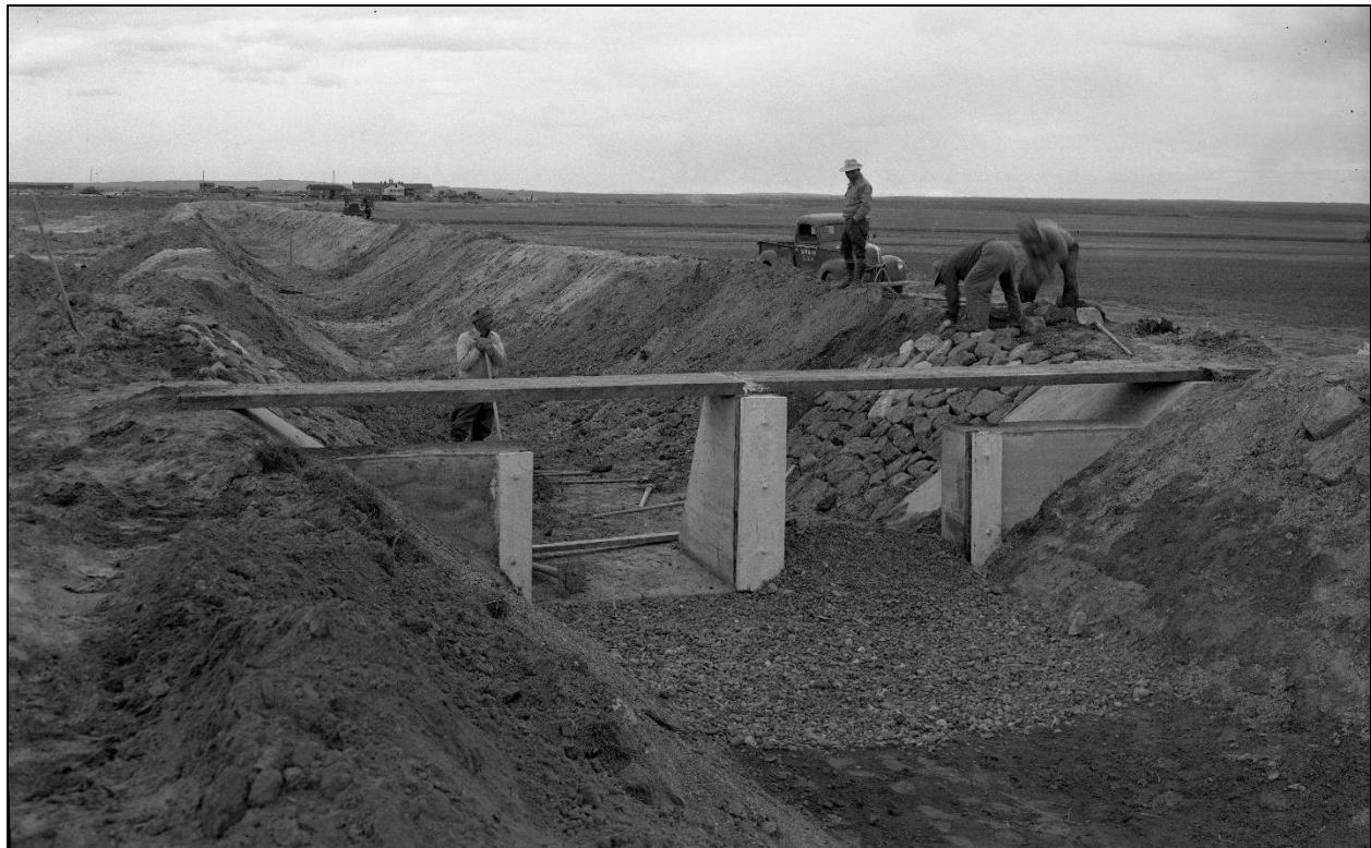
Figure 36: Irrigation ditch construction near the Minidoka concentration camp. Image available at the Denso Digital Repository, Object ID: ddr-fom-1-805 (NARA ID: 210-CMA-IC-6), Parent Collection: War Relocation Authority, Minidoka Collection, https://ddr.denso.org/ddr-fom-1-805/ . Courtesy of the National Archives.
