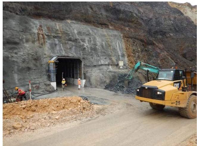
Figures 1 and 2: Portal construction at the Siana Underground Mine
