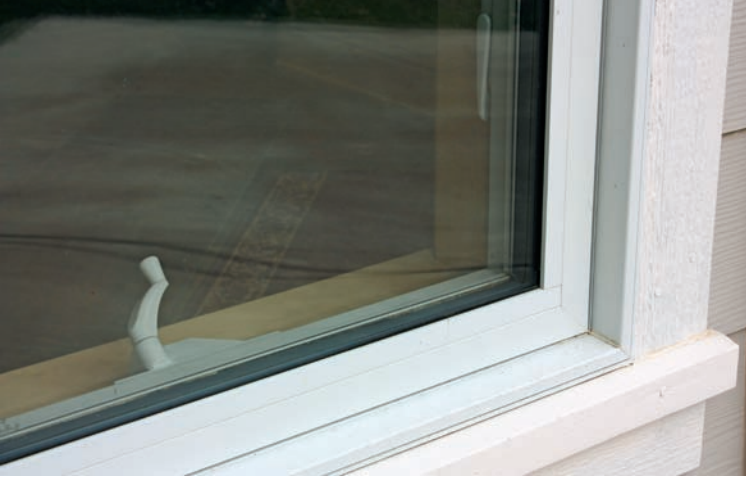
Triple-pane, argon-gas-filled windows with fiberglass frames were selected for their performance and durability.
