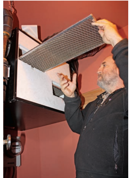
An energy recovery ventilator introduces fresh, conditioned air into the well-sealed home, with little heat loss.
