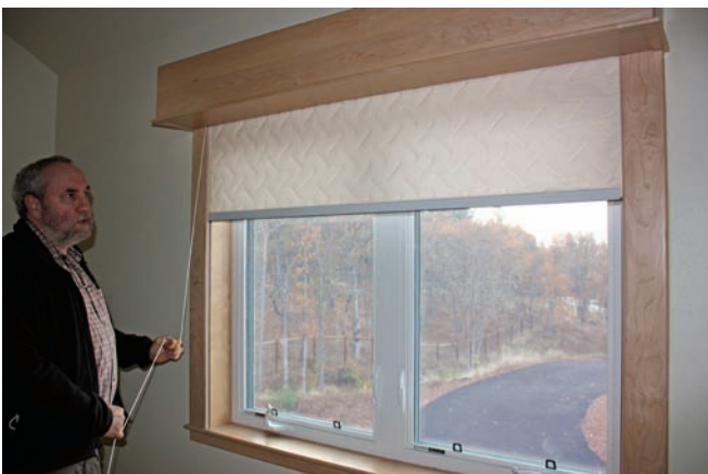
Custom thermal shades reduce heat loss through the windows.
