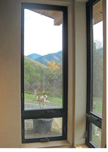
An initial appraisal mistakenly classified these high-performance, argon-gas-filled fiberglass casement windows as conventional vinyl units and neglected to recognize the value of the home's passive solar contributions to offsetting its heating loads.
