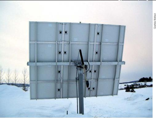
This active tracker is pointed at the brightest spot in the sky, even though there is no direct sunlight yet. The bright spot is quite low on the horizon—hence the array's nearly perpendicular position to the ground.
