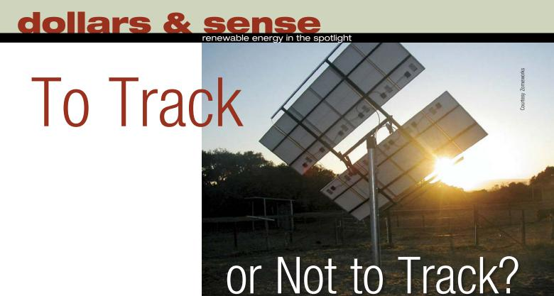
This passive tracker uses the sun—and a liquid that condenses into a gas when heated—to position the modules instead of motors, gears, or electronics.
