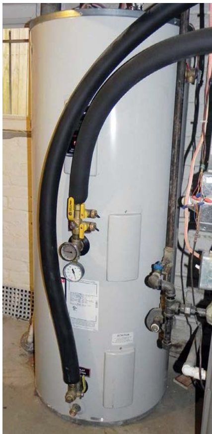
A side view of the top of the tank showing the thermometer that measures the tank's output temperature (the nearest copper pipe riser). Above it is the Honeywell adjustable mixing valve. The pink electrical cable is the 240 VAC electricity for backup water heating. The two twisted pair wires in the background connect to unused sensors (for active, not passive, systems) in the Bradford White tank.
