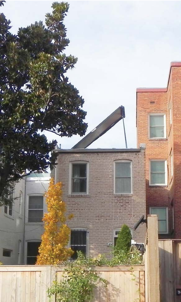
The collector has quite a presence on the modest-sized townhouse's rooftop.
