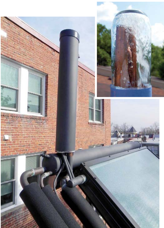
Inset: This concept model has clear glass to view the geyser’s pumping action.
