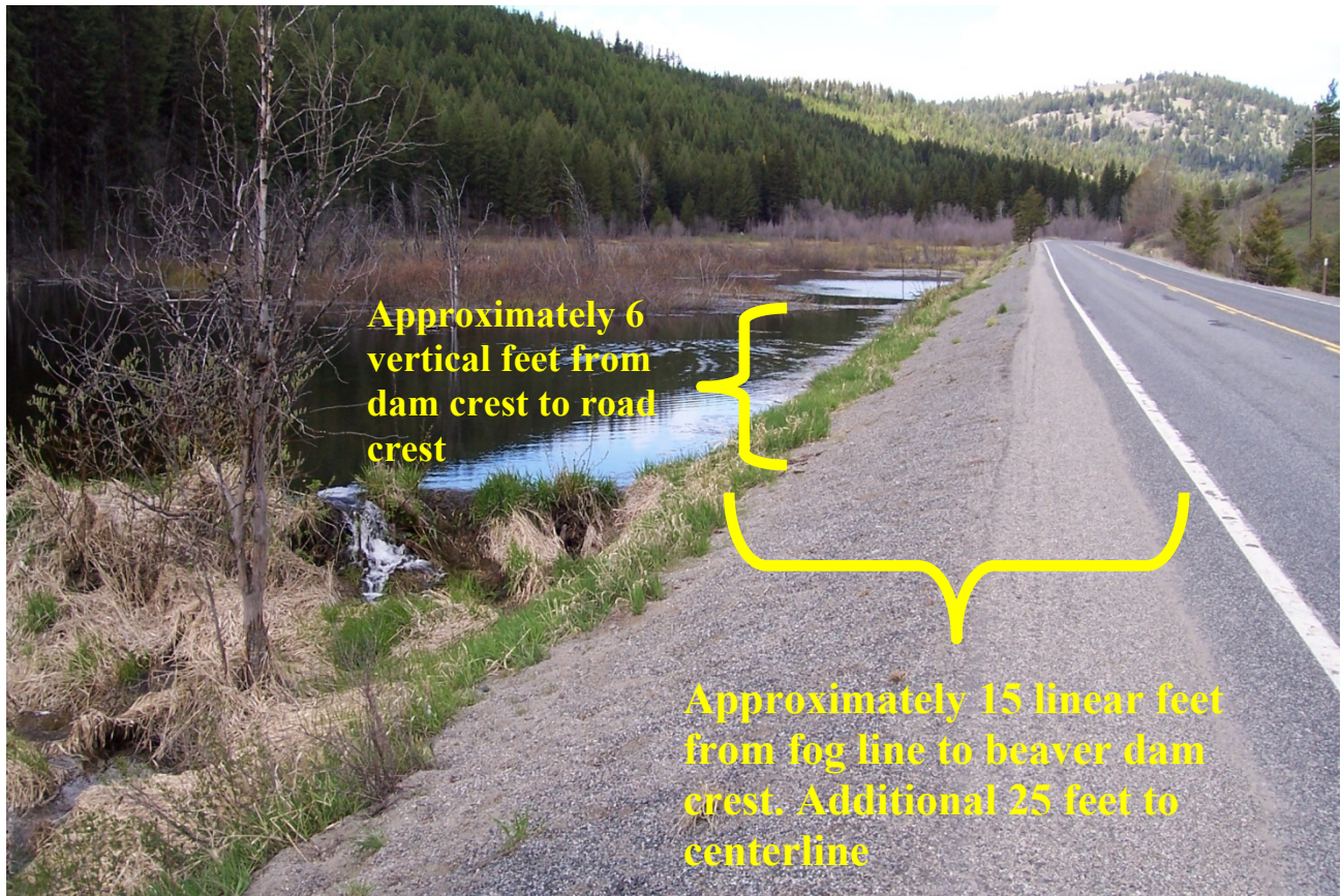
Figure 4. In this photo, the roadway is directly adjacent to a beaver dam complex on Granite Creek near Republic, Washington. The distance from fog line to the edge of the water measures approximately 15 horizontal feet, and the distance from dam crest to the top of the roadway measures approximately 6 vertical feet. Photo by Brian Walker.
