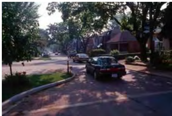
Figure 4.2k: Traffic calming neckdown or narrowing of the street, in this case, to one lane
