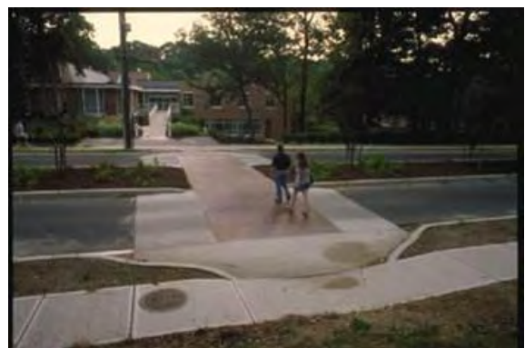
Figure 4.2m: Traffic calming: speed table or raised crosswalk
