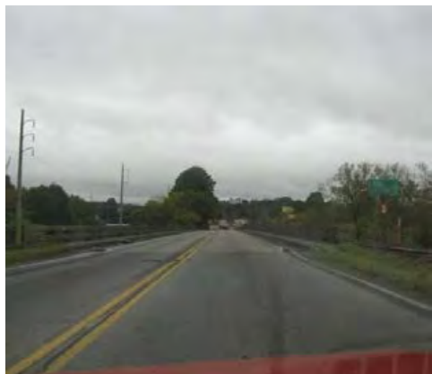
Figure 4.2f: The bridge at the Chattahoochee River would need to be resized to allow for future growth
