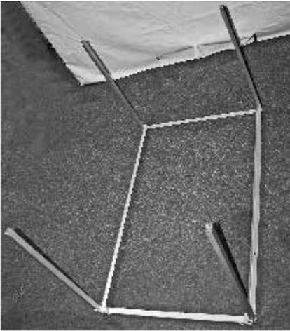
2. Attach two eave bars and two base bars to the corner blocks in the corners of the frame. The fastening strips on the eave bars should face out.
