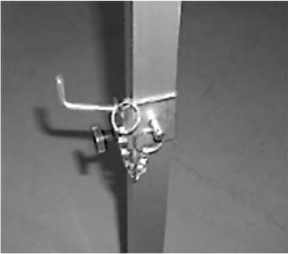
6. Attach the seat brackets to two corresponding legs and install the captive locking pin. Tighten the thumbscrew to secure the bracket.
