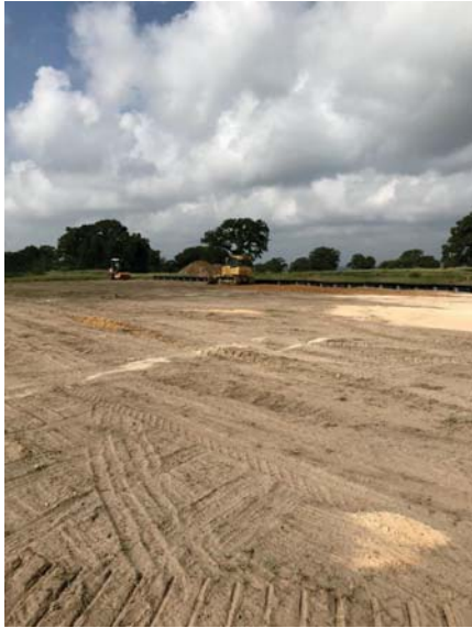
Placing base at laydown yard
