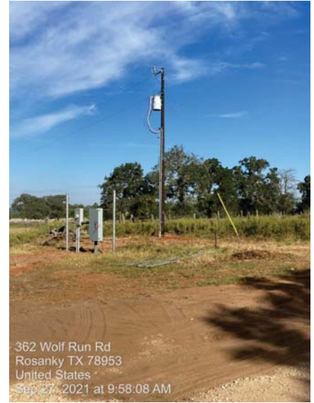
Electrical service for job trailers
