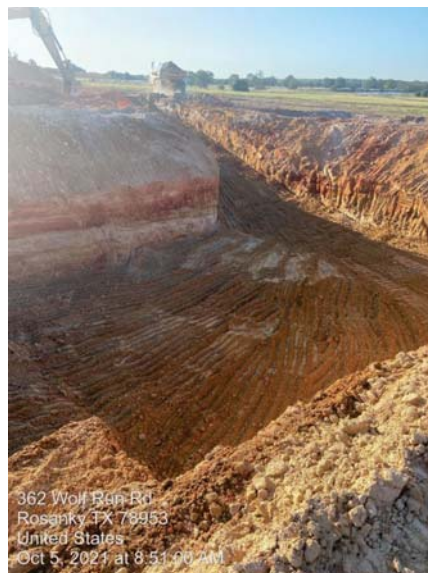
Plate settler basin subgrade
