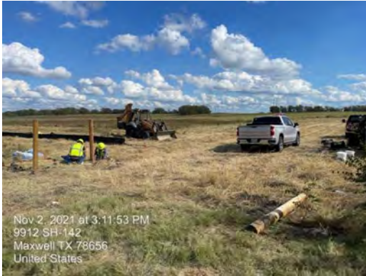
BPS – Placing fence and gate at entrance
