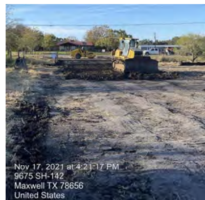
BPS – Construction entrance preparation
