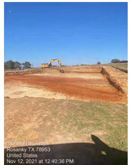
WTP/RWI - Filter Complex excavation
