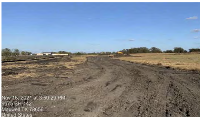
BPS – Clearing for Access Road
