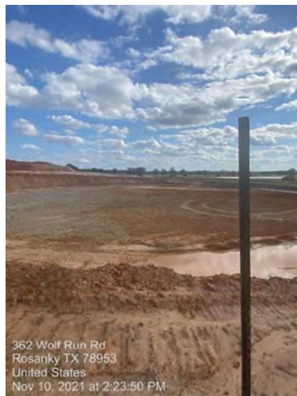
WTP/RWI - Clearwell excavation
