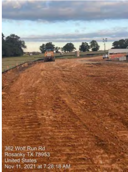
WTP/RWI - Plant Access Road
