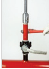
Figure 4.36. Unscrew the Drilling Machine.
