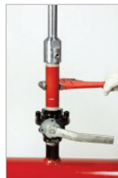
Figure 4.19. Tighten Drilling Machine
