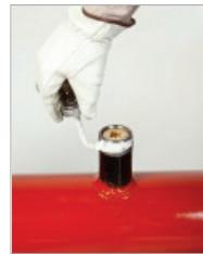
Figure 4.41. Apply Thread Paste
