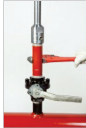
Figure 4.50. Tighten Drilling Machine
