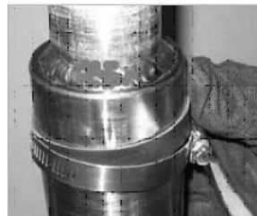
Figure 5.9. Secure Extension Base
