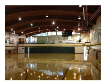
**Before** – At 28 feet this gym had only 11 foot candles of light at center court using (24) 400 watt metal halide lights.
