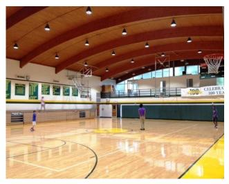
**After** – Using (30) SONARAY™ 250 watt Delta high bay lights, center court measured 91 foot candles at 28 feet.
