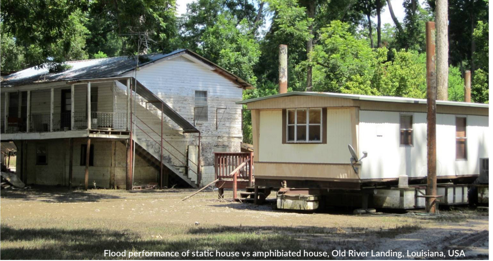
Flood performance of static house vs amphibiated house, Old River Landing, Louisiana, USA
