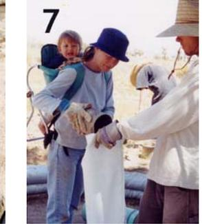
4) Place the door away from wind and water. 5) Dig the foundation trench 30 cm (12") deep. 6) Level and compact. (The foundation will be 2-3 completed bag rows.) 7) Place the bag in the trench, fold the end under to close, and start filling upright like a short column.
