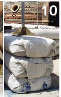
8) Always put in 2-3 cans of earth and shake to the end. 9) Use gravity's help by sloping the bag on your leg, and walking backwards as it fills - do not strain. Let the bag fill as full as possible and check the position with the compass tool. 10) Twist and tuck under the bag ends to close.
