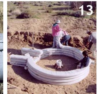
11) Compact the filled bag as hard as you can using a tamper, to make a smooth, solid, uniform block. Only compacted earth becomes strong. 12) Attach continuous barbed wire - 1 wire for domes up to 4m (12 ft), 2 wires for bigger. Where breaks occur, overlap the wires by 2ft. (65 cm). 13) Continue coiling bags.
