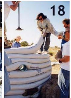
**16) Pre-cut bags for a doorway knock-out panel. Stabilized earth must be cut after tamping at every row - don't let the cut stick back together. 17) Punch out pre-cut panels to open after a min. of 5 rows, or when the dome is completed. 18) Insert pipes for windows sloped to outside for rain.**
