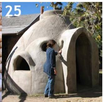
**22) Plaster the exterior before bags disintegrate and 23) waterproof with locally suitable materials to resist moisture and erosion. 24) On top, finish with a water-resistant cement/lime plaster such as Reptile (cement or lime mud-balls) layered from bottom to top, or 25) a smooth cement or lime plaster finish.**
