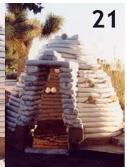
**19) Coil upper rows, but don't stand on the wet bag. 20) Fill and place bag above the row below and work it inwards to meet the compass circle. Tamp the bag with gentle slope to outside. 21) Add an arched entry (door vault) to the opening to buttress and protect the entrance. Entry is arched or sloped, short or tall.**
