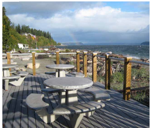
Made from recycled plastic lumber, the deck also used most of the existing footings and substructure from the restaurant building that originally occupied the site.
