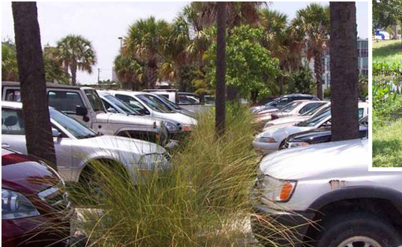
Experiments with vegetated swales and pervious pavement in the parking lot (left) significantly reduced runoff and protected water quality. Runoff from the queuing garden was directed to a small pond (above).
