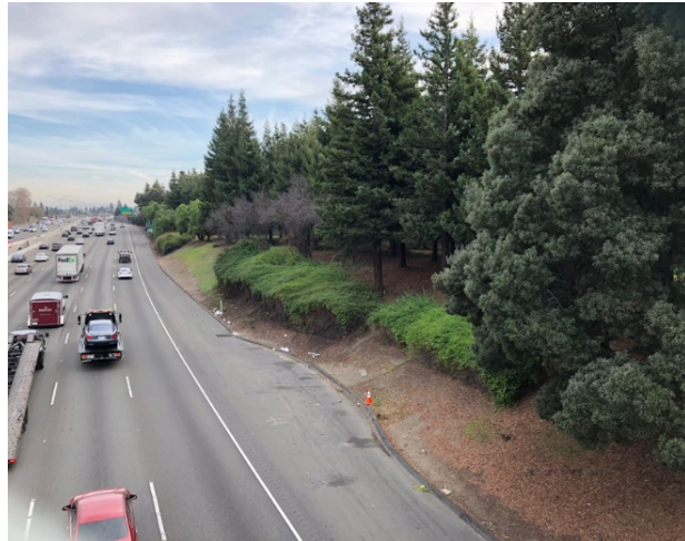
Partial view of area where trees will be removed. Trees will be removed on the southbound side of I-880 both north and south of Hacienda Avenue.
