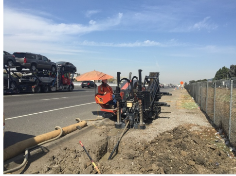
Directional boring on southbound I-880
