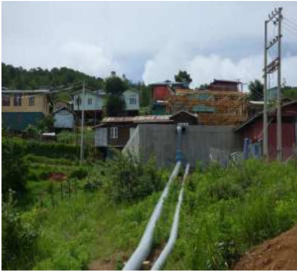
Timit tilak mi tipeknak ti pipe le tikhonnak ti-inn, sipin nih nawl an chuah tik in Hakha khuachung tipeknak (Credit: Carl Middleton)
