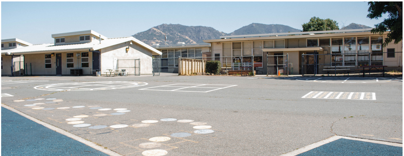
Extensive asphalt and rubber surfaces are typical in California schoolyards. These materials heat up in the sun and expose children to high temperatures.
