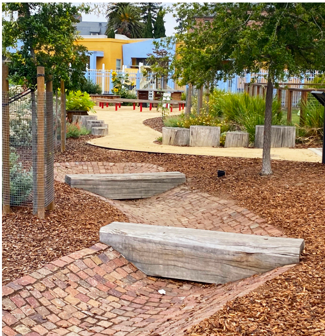
A bioswale (left) collects and stores stormwater runoff. Planting shade trees (right) is an excellent way to reduce temperatures on school grounds.
