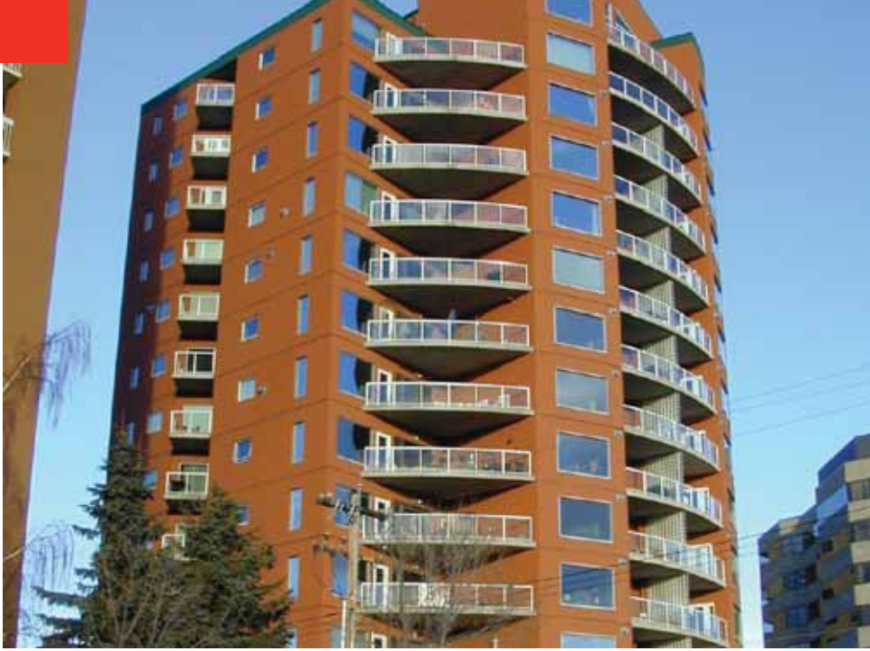
Figure 1: Southwest Elevation Grandin Green Building
