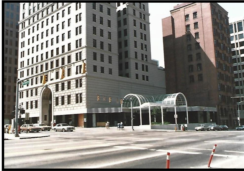
1985 Southwest Corner of Broad and High
