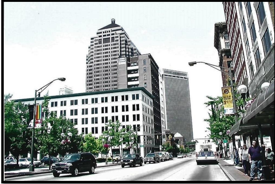
2005 Photo North on High from Elm
