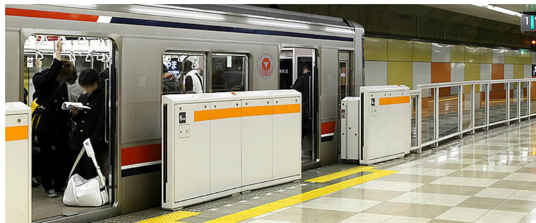
Platform screen doors of Ookayama Station, Tokyu Meguro Line
